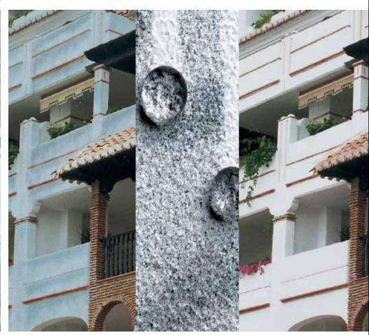
**The problem with conventional exterior paints:** The soiling of the façade becomes increasingly visible over time. On weather exposed sides in particular, microorganisms find an ideal environment for colonization in the form of adequate moisture and nutrients from dirt deposits.
