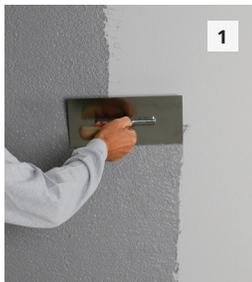
**1** Using a stainless steel trowel, apply Stolit 1.0 and trowel off to aggregate size. Only apply finish to the area that will be textured immediately.
