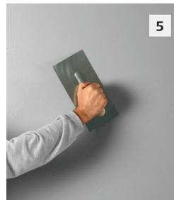
**5** To create the texture, hold the trowel at a steeper angle. Trowel in a crisscross pattern to produce a finely rippled texture. Leave the surface to dry.
