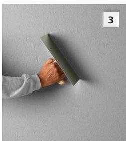
**3** Knock the tips off the dried finish using the edge of the stainless steel trowel. Blow/brush all loose particles from surface.
