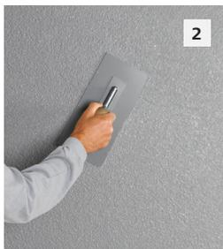
**2** Float the freshly troweled finish in figure eight movements using a plastic float. Always remove any excess finish paste from the plastic trowel. Leave the surface to dry.
