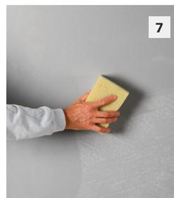
**7** Wash the finished facade with clear water or carefully dust off dry. Optional: apply Sto Clear Coat Sealer of desired gloss.
