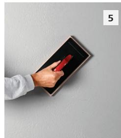
**5** When the surface of the Stolit Milano starts to dry, float the entire surface with a slightly damp Sto-Rubber Sponge Float in a nondirectional manner. Leave the surface to dry.
