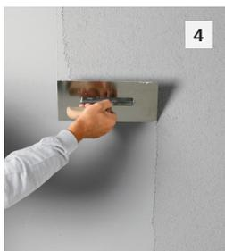
**4** Using a stainless steel trowel, apply a thin coat of Stolit® Milano as a second layer to the dry Stolit 1.0. Only apply finish to the area that will be textured immediately.
