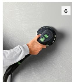
**6** Once completely dry, sand the surface within the next day using a power or manual sander with a dry abrasive paper of P80 - P120 grit until the desired surface texture has been achieved.
