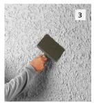
Immediately afterwards, partially smooth the textured peaks of the finish while it is still wet using the knockdown trowel in a crisscross pattern, in no particular direction, applying light pressure.
