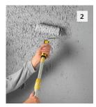
Immediately texture the finish while it is still wet using a texture roller in short strokes and in a crisscross pattern across the area, working from bottom to top.
