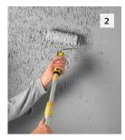
Immediately texture the finish while it is still wet using a textured roller in short strokes and in a crisscross pattern across the area, working from bottom to top. This creates a very coarse, sharp-edged texture.
