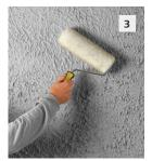
Leave the finish until it is dry to the touch. Level the sharp-edged tips of the finish using a dry, short-pile roller. Guide the facade roller across the finished surfaces in a crisscross pattern, in short strokes, applying only light pressure. Rolled, coarse texture, partially smoothed.
