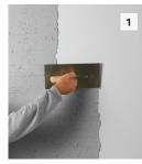
Apply the finish to the uniform primed surface, using a stainless steel trowel, to a thickness slightly over the aggregate size. Only apply finish to the area that will be textured immediately.
