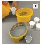
Dilute StoTique with water up to the maximum amount as indicated in the Product Bulletin. Stir StoTique frequently during its application. Note: if less water is used, StoTique will be thicker. This may be preferred and more suitable to created desired effect.
