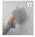
One application technique is to evenly apply StoTique in patches using a spray bottle. Apply StoTique using a brush, roller or sponge. Take care not to apply them in a straight line, particularly in areas such as scaffolding platforms.
