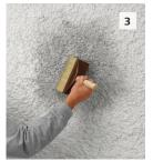
Immediately smooth StoTique using a brush, sponge or a cloth. Leave the spots from the first application cycle to dry thoroughly before starting the second application.
