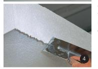
Once the basecoat is dry, apply the finish. Remove any protruding finish from the edges.
