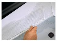
Apply basecoat at the return area. Align the Sto Drip Edge Profile, press it into place, and fully embed it in the wet basecoat.
