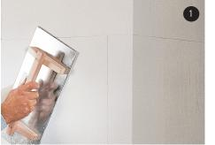
At building corners, the insulation boards should be interlocked. Saw off any protruding insulation boards at external corners. Rasp the insulation boards to ensure that they are even.
