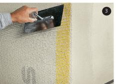
When applying the surface reinforcement, guide the Sto Mesh into the corners. Overlap the Sto Mesh corner bead standard by at least 4 inches. Cut off protruding
